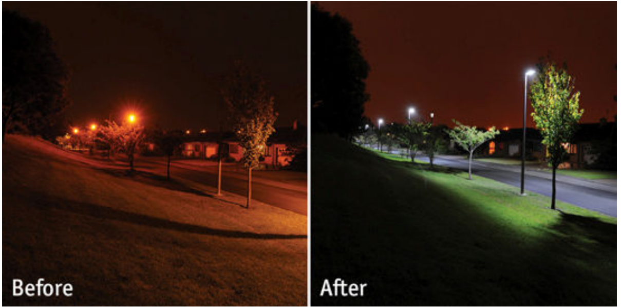
3/18 Pictures of a trial in Middlesbrough showing Before with SOX Lighting and After with LED's.
